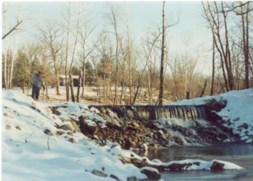
The restored dam in January, 1993
